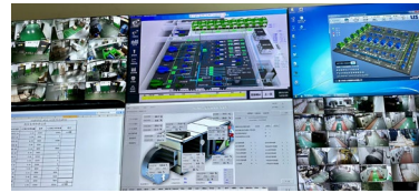
>> TPV Fuqing Visualized Digital Energy Monitoring System
